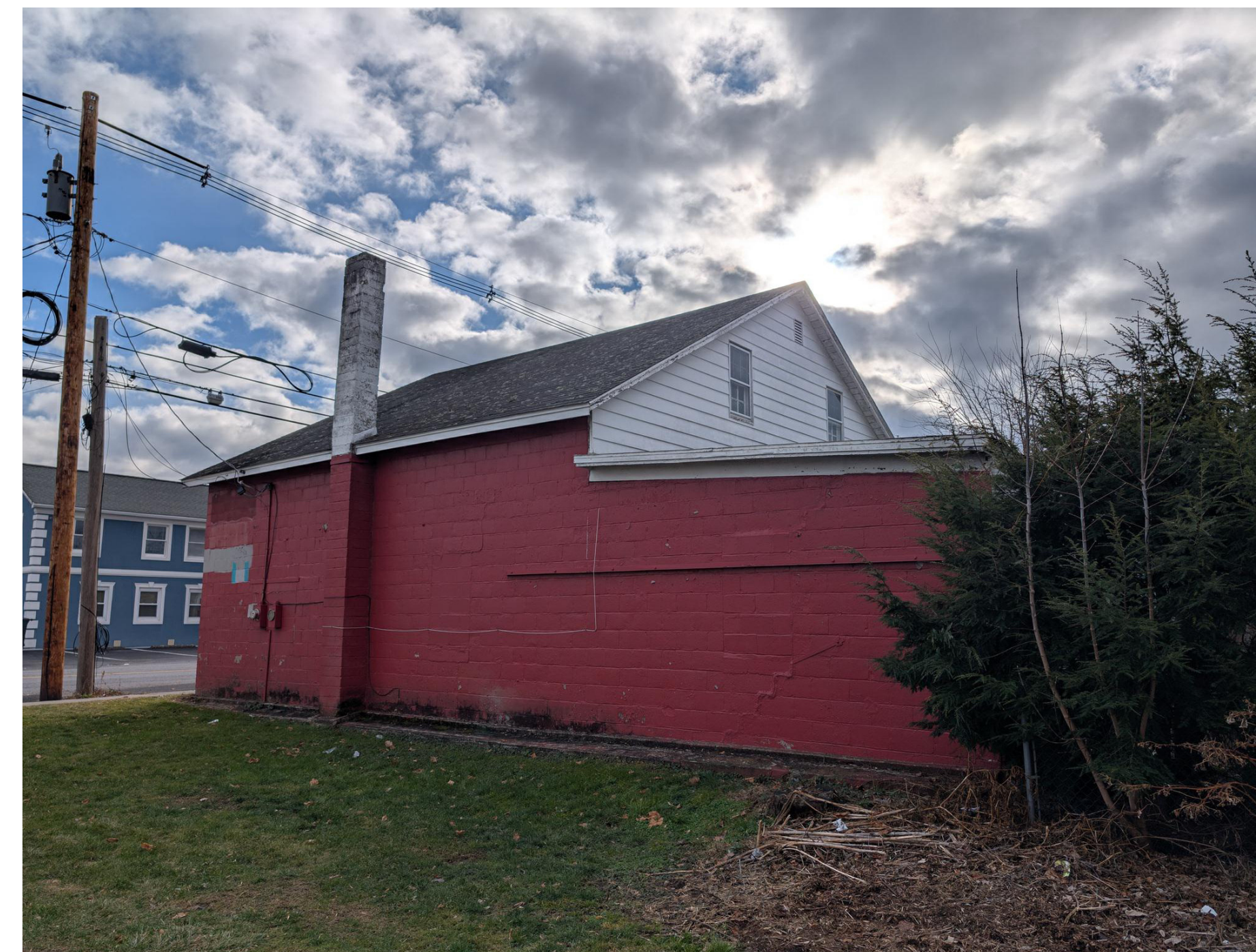
4 EXISTING BACK PHOTO 3EP1.0 NO SCALE
