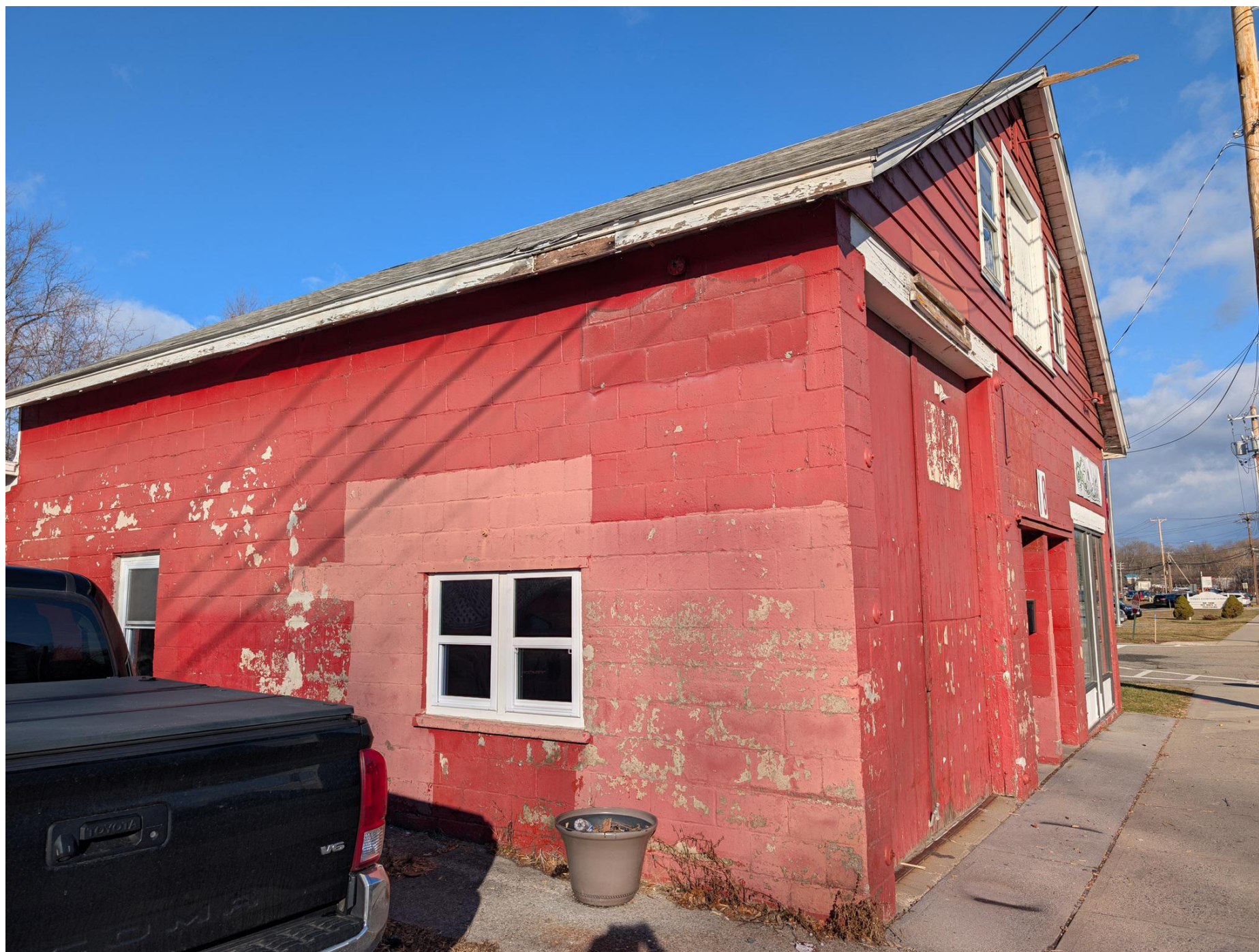
3 EXISTING LEFT PHOTO 3EP1.0 NO SCALE
