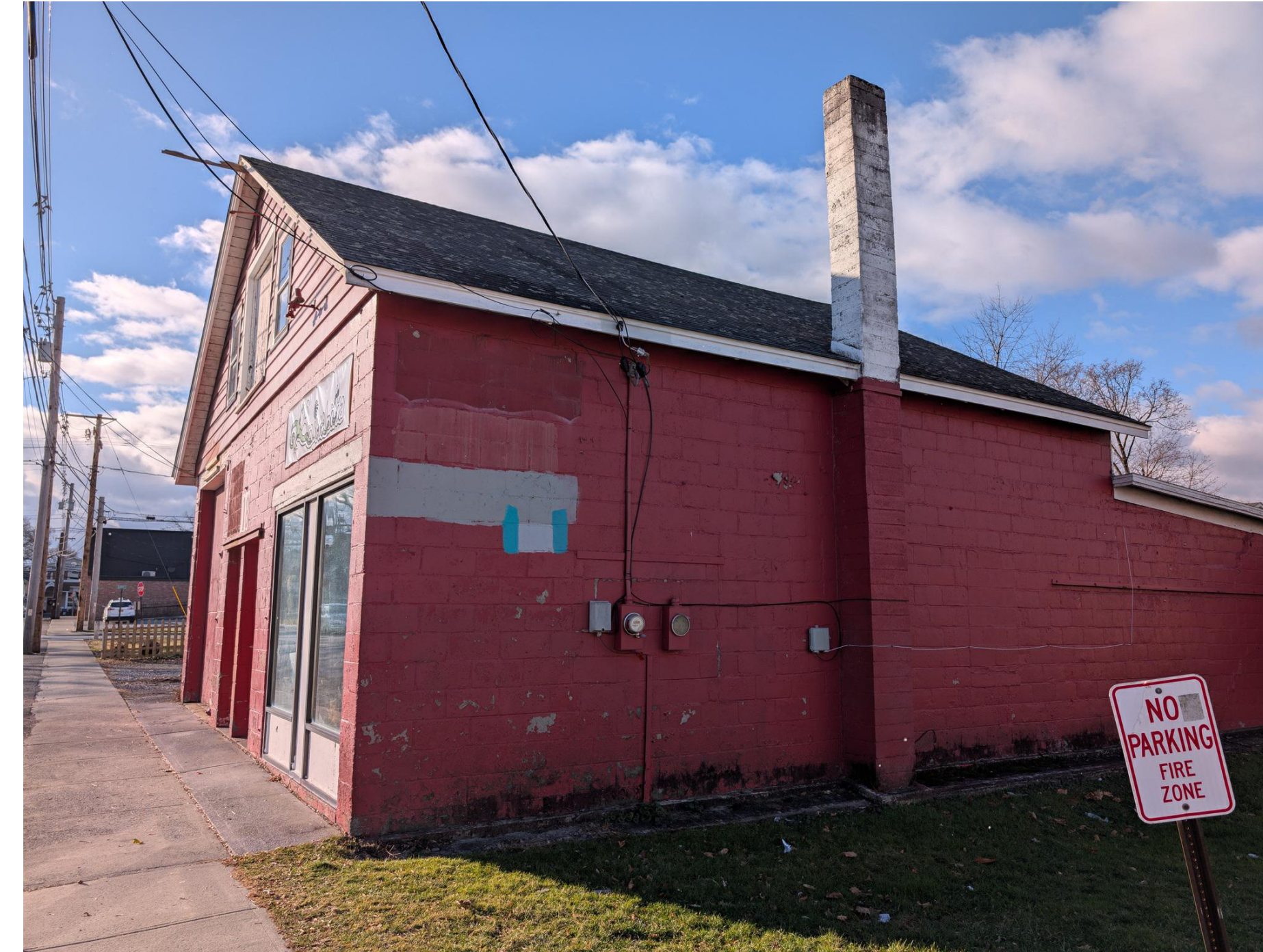
2 EXISTING RIGHT PHOTO 3EP1.0 NO SCALE
