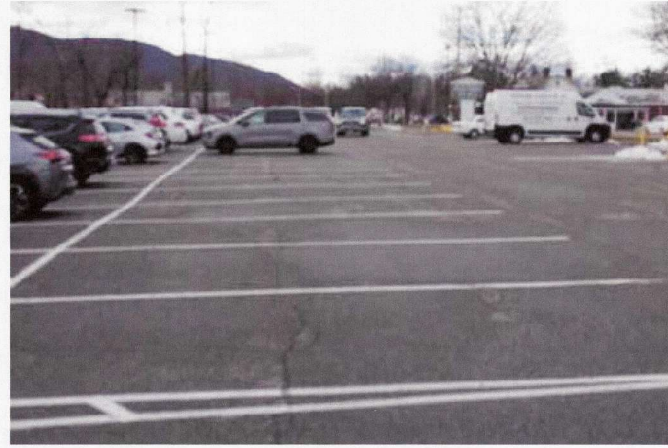
DATE: 12/19/2024 TIME: 10:15 AM FACING SOUTH WEST
