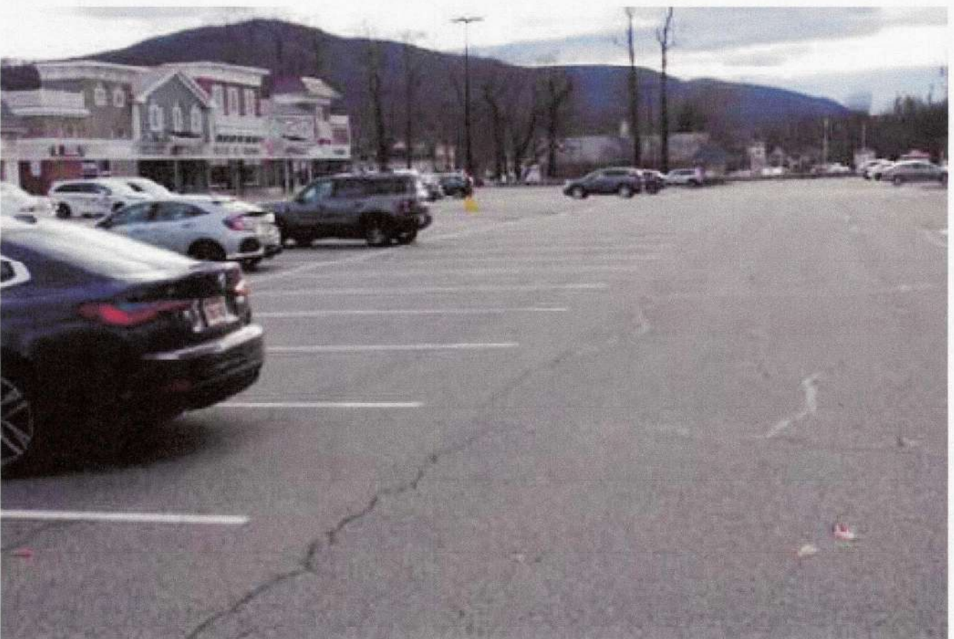
DATE: 12/30/2024 TIME: 2:06 PM FACING SOUTH TO PLAZA
